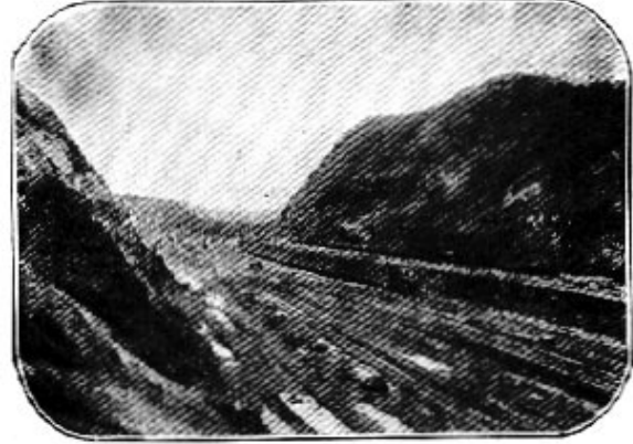
PANAMA CANAL — CULEBRA CUT
