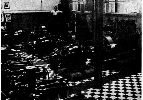
300 Horsepower Is Developed by These 4 Diesel Engines.
