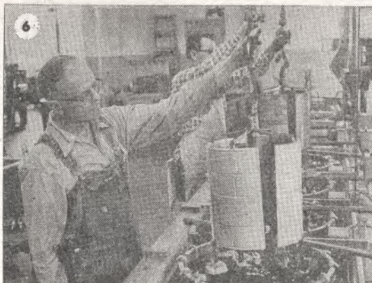
Coating plates with nickel
