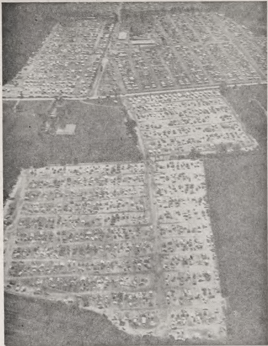
Aerial view of the trailer camp
